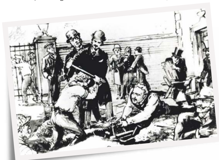
Ferranti's chisel test, below, demonstrated how he had effectively earthed 10,000V
